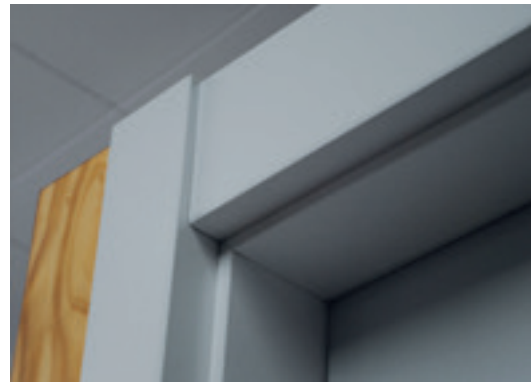
Finishing top of the kit installed
