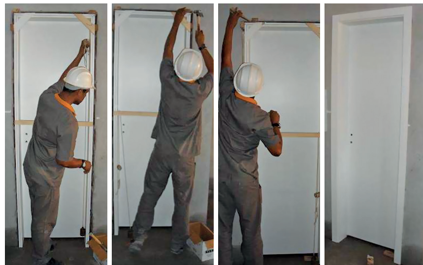
Installation process of kit at the construction site.
